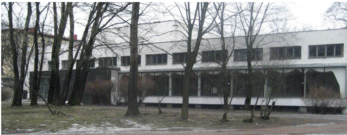
Figure 2 – North view through trees, 2012.
