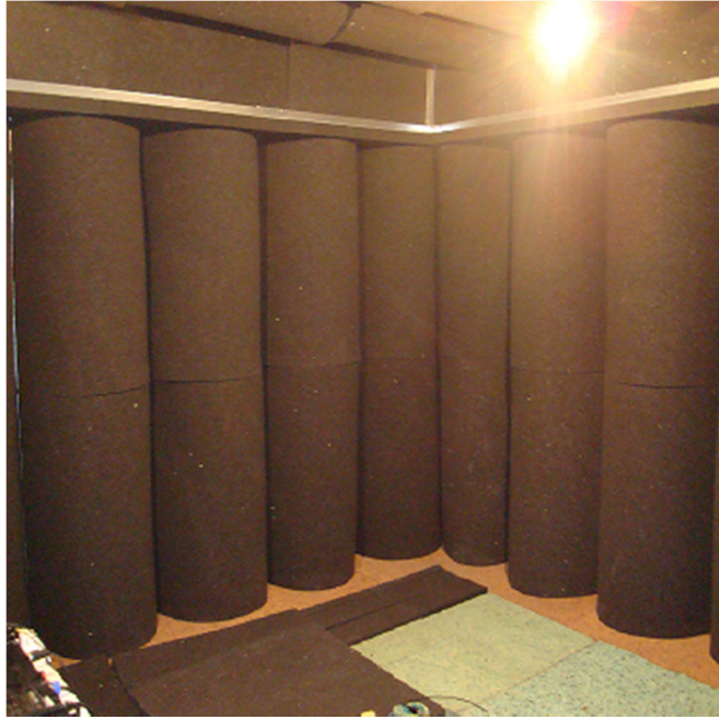
Figure 3 – Quasi-anechoic test chamber for the noise barriers.
