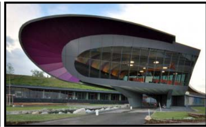
Figura 3. Administration Building for ZMS. Alemania.
