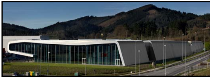
Figura 2. Edificio AIC Automotive Intelligence Center. Bilbao, España
