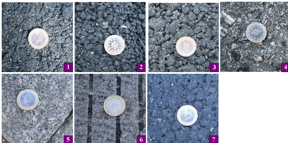
Figure 4 - Pavements analyzed in this study. 1- dense asphalt (PA) (new), 2- gap graded asphalt rubber (GGAR), 3- rough thin layers (RTL), 4- dense asphalt (DA) (old), 4- dense asphalt (DA) (old), 6- cement concrete (CC), 7- rough asphalt rubber (ARR).
