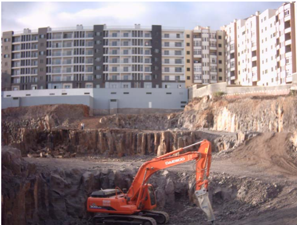
Figure 3 - View of the Madeira works site
