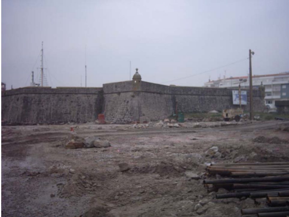
Fig. 2 – Blasting site, Fort and houses behind on the portuguese coast.
