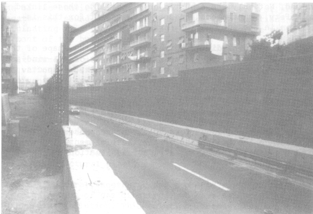
Fig. 1 - Antinoise barriers under construction near Railway on the Highway "A10"
