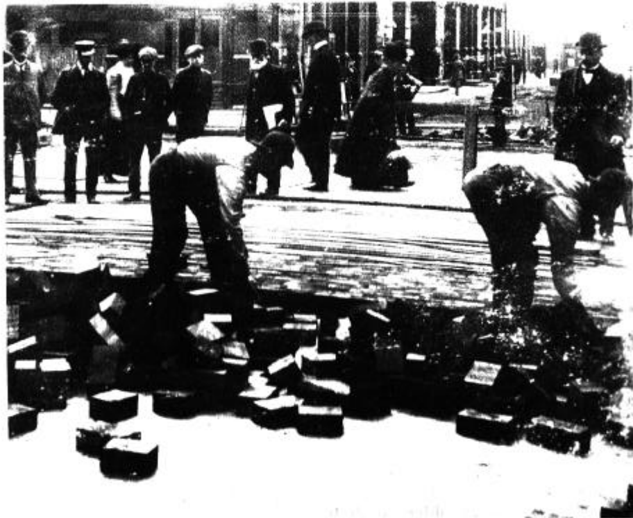
Fig. 1 Laying of wood blocks in a street in Oslo around 1914.
