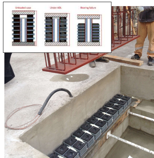
Figure 11. Installation of the VHS (very high stress) bearings with integrated failsafes.
