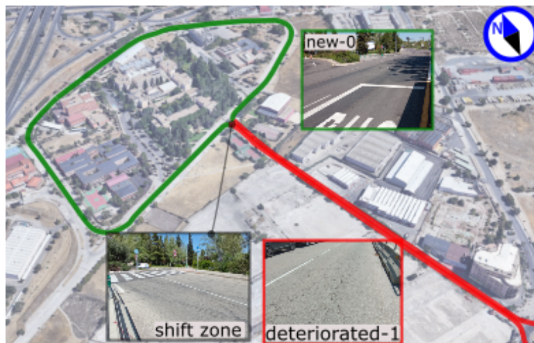
Figure 2: Actual road status on experimental route.
