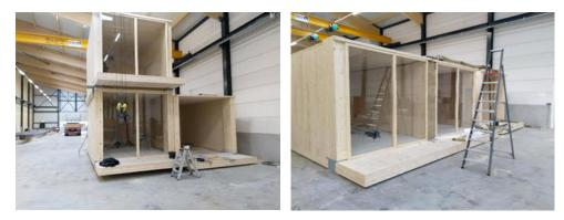
Figure 3. The CLT modules in the vertical arrangement (left) and in the horizontal arrangement (right).
