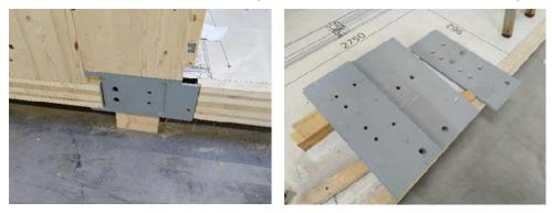
Figure 4. The floor steel element (left) and the steel connection plates (right).
