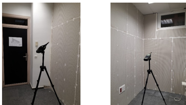
Figure 13 – Control room with the proposed solution installed
