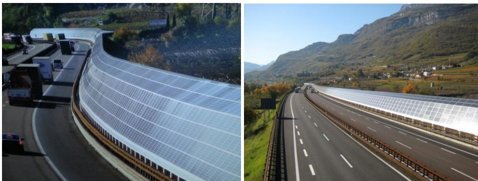
Figure 6: Noise barrier to produce energy [8].
