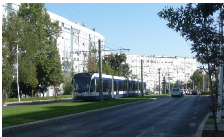
Figure 4. Almada light rail.
