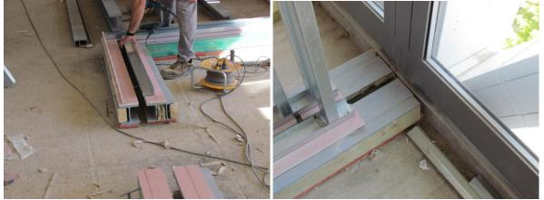
Figure 3 – Details of the double wall construction between rooms, with an underlying anti-shock material for additional sound insulation.
