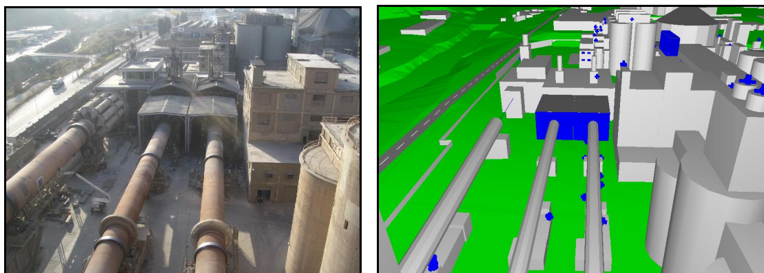
Figure 13 – View of the three cement kilns at present: photo (left) and model (right).
